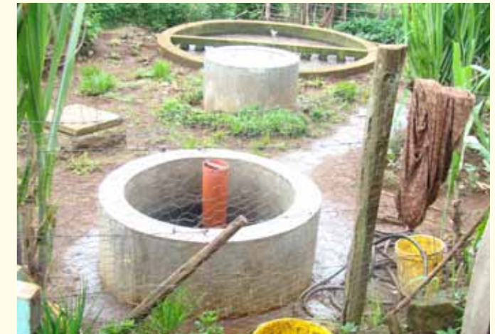
An installed Biogas unit in one of the beneficiary's home.
