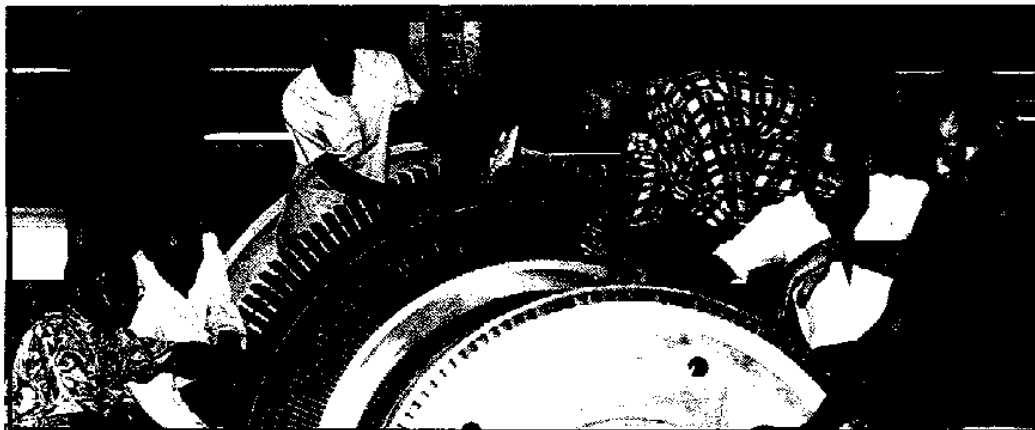
Turbine No. 6 at Kipevu Power Station was overhauled to enhance generation capacity.
